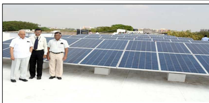
MNRE / TEDA / KCT Sponsored on Grid 50 kW Solar Power at KCT – EEE Block
