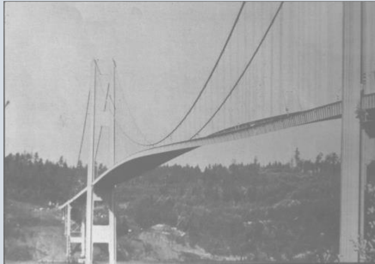
Tacoma bridge rotating about its body axis
